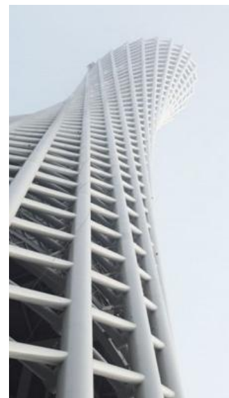
Figure 14: Torqued ellipse by Richard Serra at Bilbao Guggenheim Museum (left) and torqued ellipse structure in the Canton Tower in Guangzhou (right).
