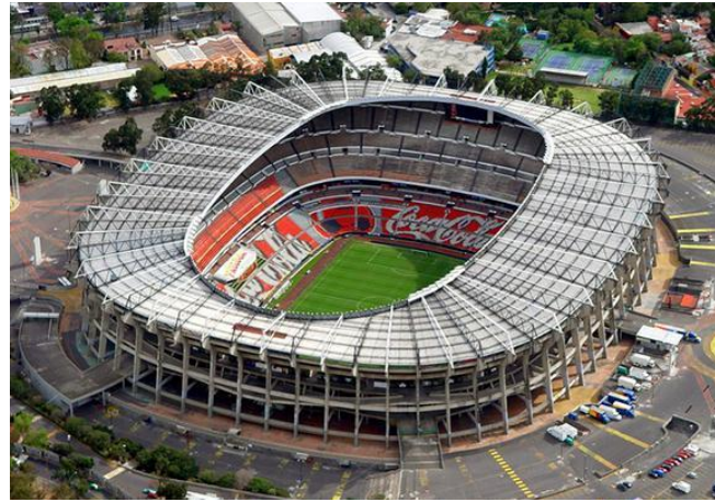
Figure 13: Two examples of superellipses: the project of Z15 Tower, the future tallest building in Beijing (left) and the Aztec Stadium, constructed for the 1968 Olympic Games in Mexico (right). Many sport stadiums feature the superellipse in their floor plans.
