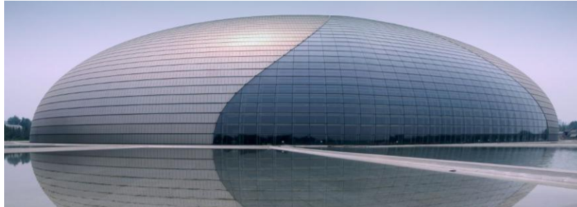
Figure 11: The National Centre for the Performing Arts, usually called The Egg, is an ellipsoid dome of glass and titanium surrounded by an artificial lake. Designed by Paul Andreu, Beijing, 2007.
