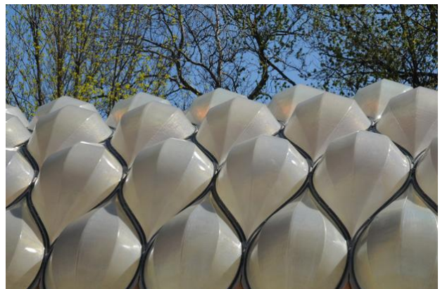
Figure 4. Nested Fiberglass domes. Image © Studio Gang Architects.
